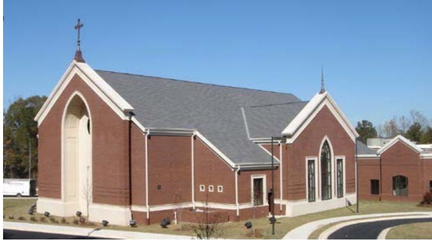
[Image: St. Michaels, 2011; Source: http://www.millermizeprecast.com/galleryLarge.cfm?ID=32 ]
